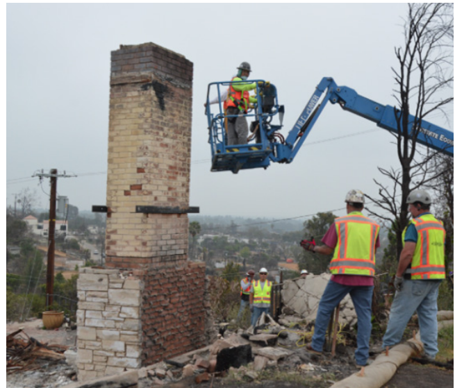
Photo 7 After Palisades Wildfires, Only Brick and Masonry Chimneys Remained Intact
