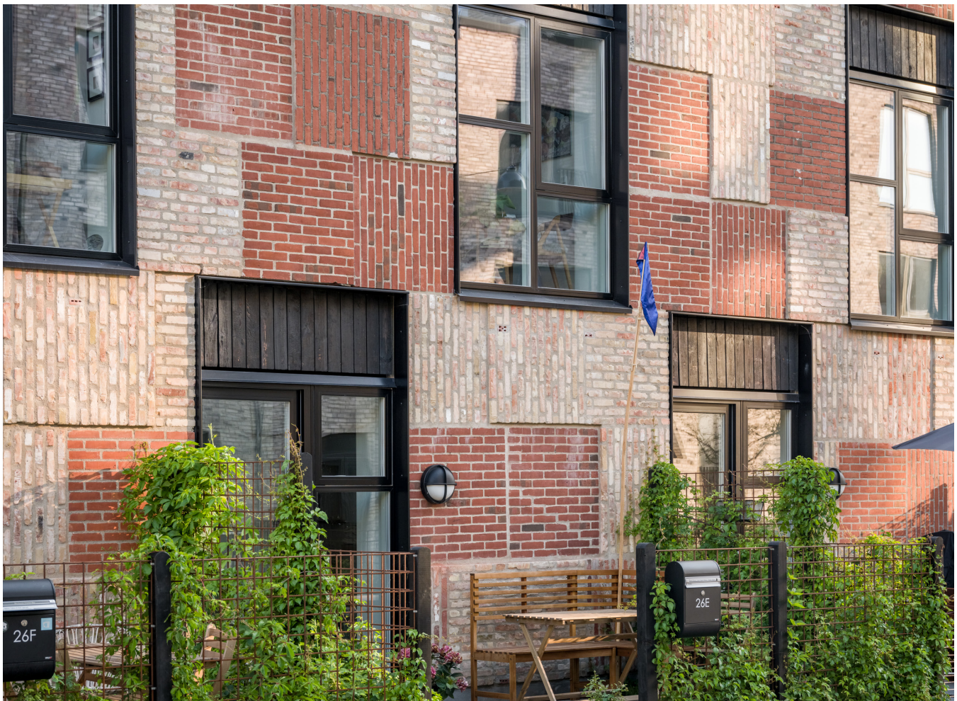
Photo 3 Panelized Reclaimed Brick Masonry (Resource Row)
