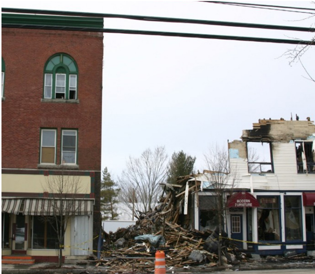
Photo 6 Brick Building Undamaged After Fire Destroys Neighboring Building
